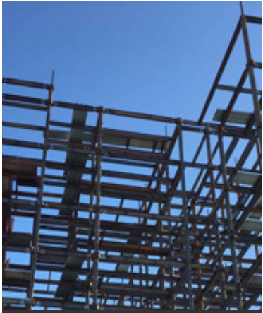
Selma Tommie Hotel: 9 story a commercial building consists of 212 Hotel guest room with ground floor courtyard, roof top pool and roof deck and 173 parking stalls Selma Tommie hotel is an XR200 project with 560 nodes and 450 ton of steel.
