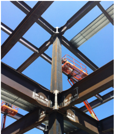
SV6 Data Center: To solve the problem of future configurability, upgrades, and mechanical system routing, the lack of shear walls in this instance allowed for a fully open and reconfigurable floor plan. The ConXL System also delivered a solution for the highly concentrated floor loadings (275 psf) required with unparalleled structural efficiency.
