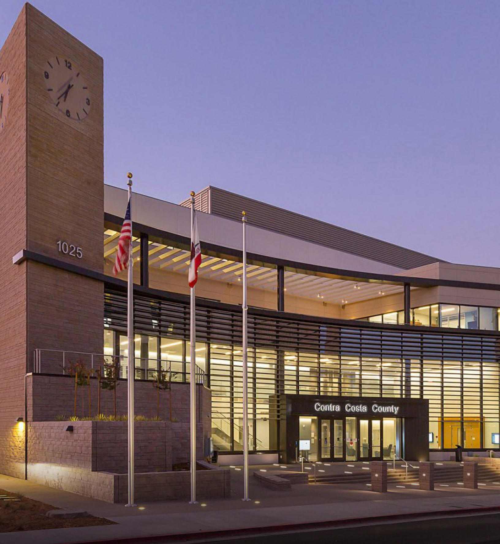
Contra Costa County Administration Building
